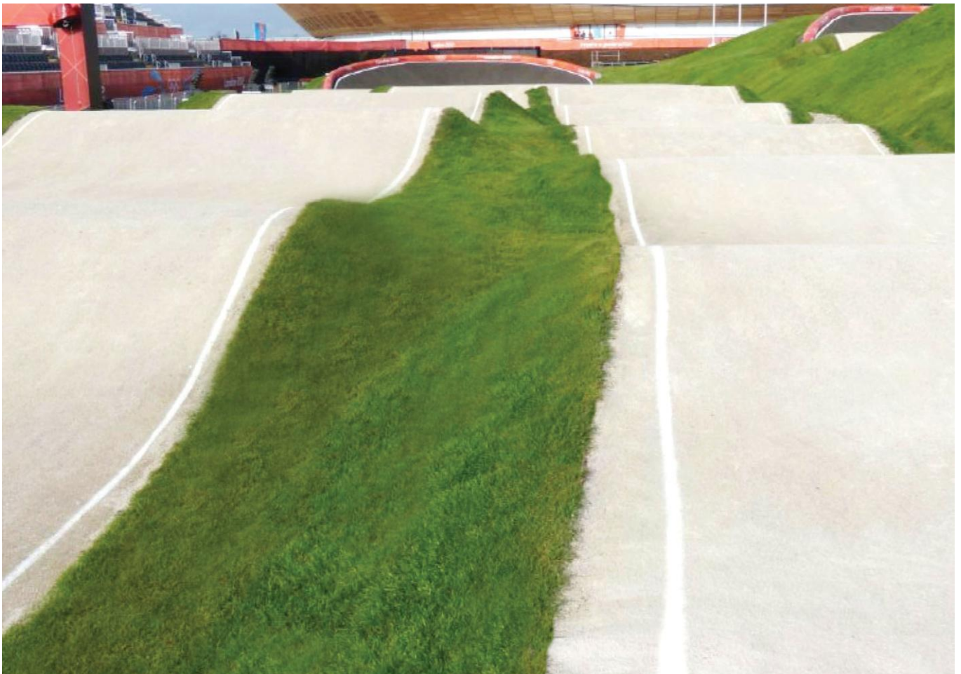
Straight 3 London 2012 olympic track (UK)
